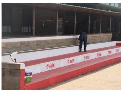
Renovation of the Terraces by Airtel
