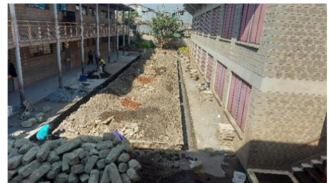
Grade 9 classrooms construction at St. Elizabeth
