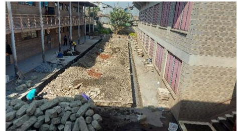
Grade 9 classrooms construction at St. Elizabeth
