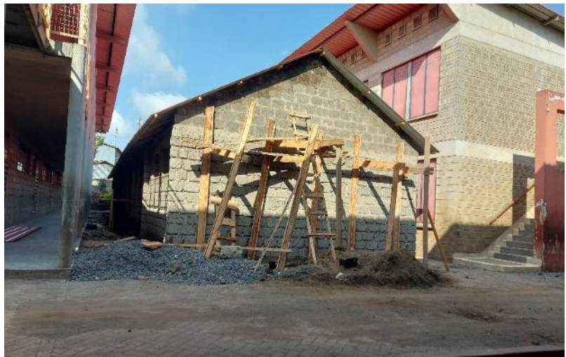
Under construction St Elizabeth Grade 9 Classrooms
