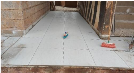
Tiles repair at St. Bakhita primary school
