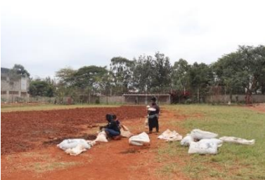
Refurbishment of the fields underway
