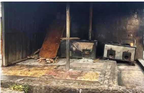
Before the repairs
