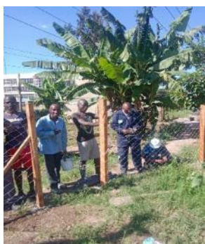
Charles and the carpentry boys fencing the MIRC gardens
