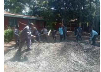
The carpentry boys spread out the blue metal gravel
